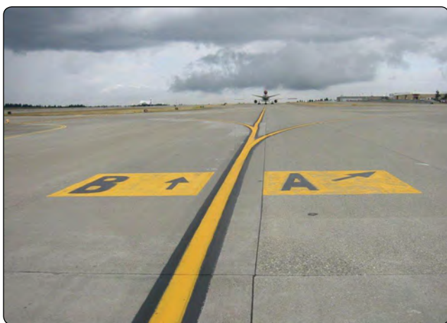
Figure 14-19. Surface painted taxiway direction signs.
