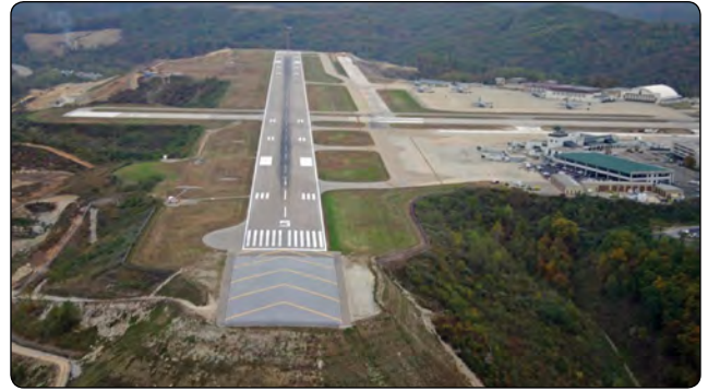
Figure 14-55. Engineered material arresting system (EMAS) located at Yeager Airport, Charleston, West Virginia.
